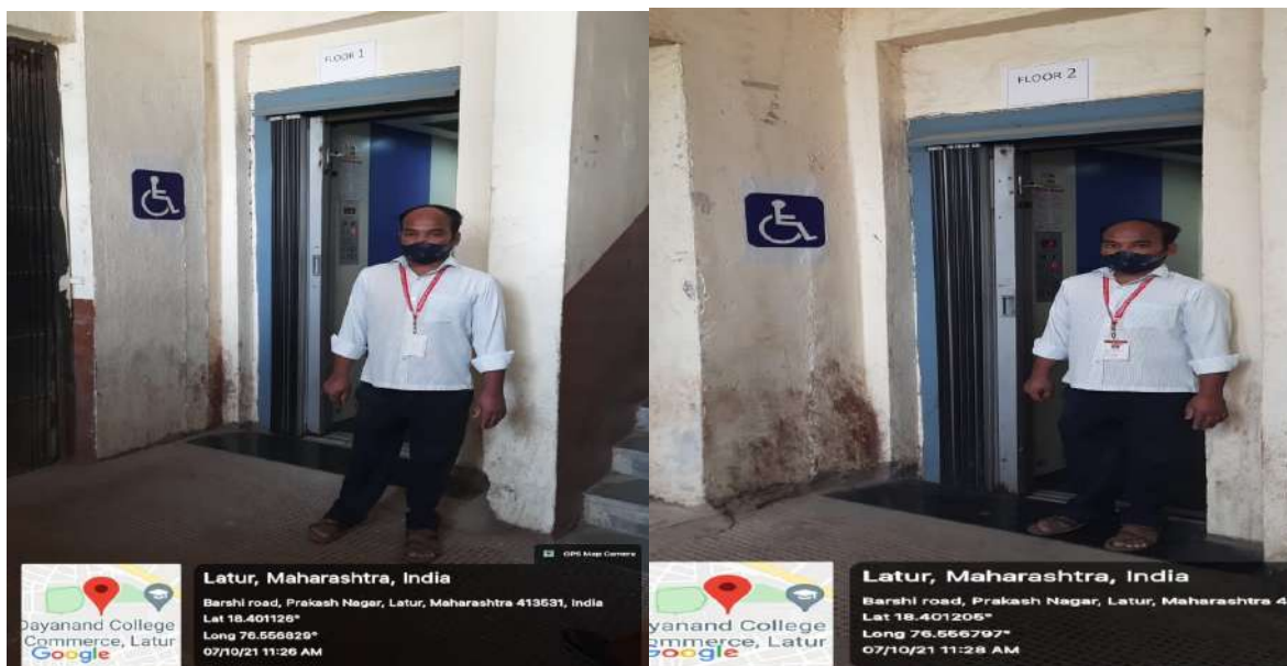
Facility of lift
