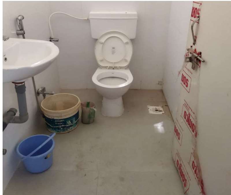
TOILET FACILITY FOR DIVYANGEN
