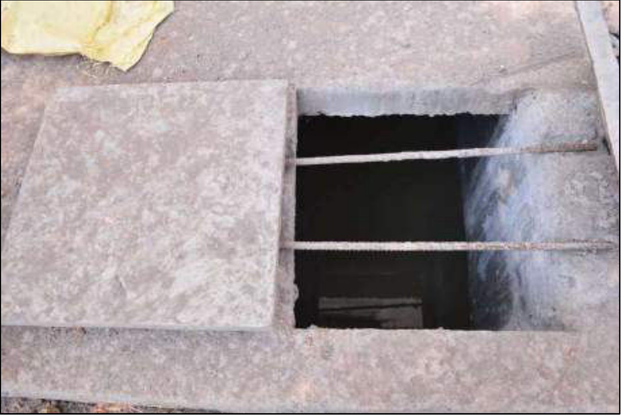
Figure 12: Rain Water Harvesting
