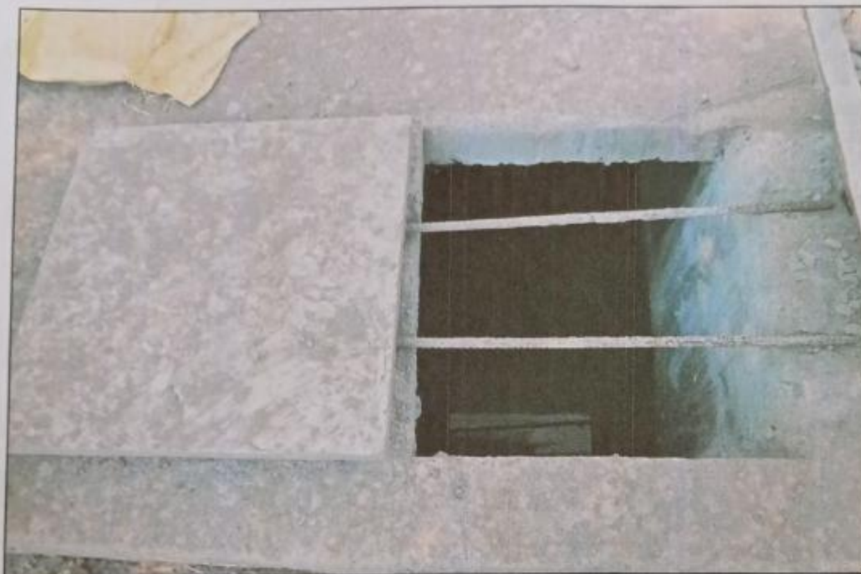
Figure 12: Rain Water Harvesting
